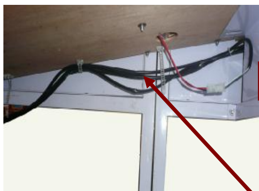
The extra light belt is wrapped with nylon tape
