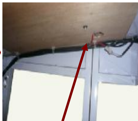
The extra light belt is wrapped with nylon tape
